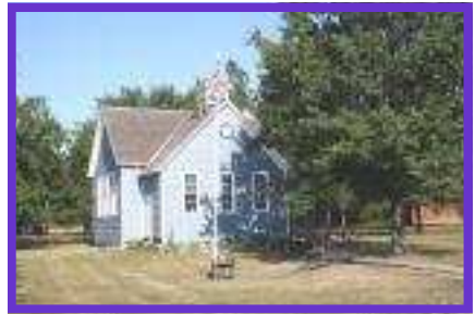
Our little schoolhouse is undergoing some much needed renovations. Thanks, Claude and Bob!
